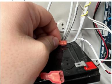
5. Once the battery is reconnected, close the alarm panel and the battery trouble will go away (Sometimes you might need to arm and disarm the system to clear the trouble)
