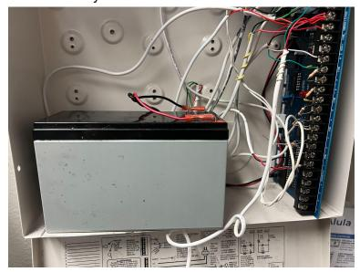
3. Carefully remove battery leads. Sometimes they do get stuck and you can give it more force to pull it off
